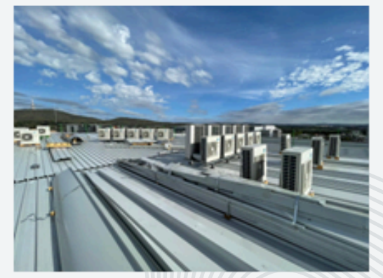
Air conditioning replacement, Parramatta
