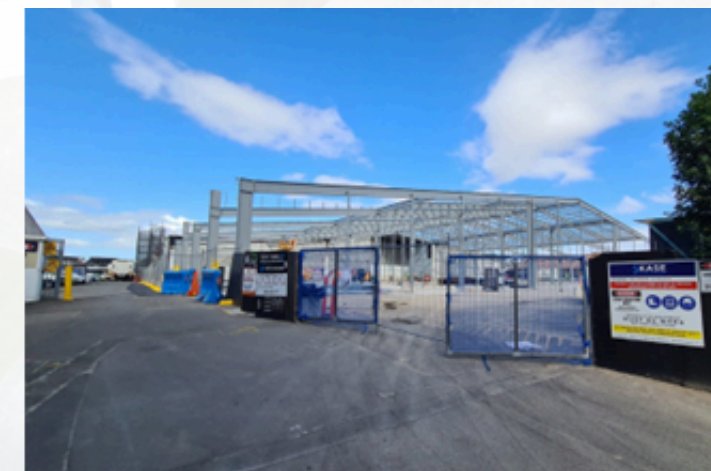
Warehouse fire rebuild, Alexandria
