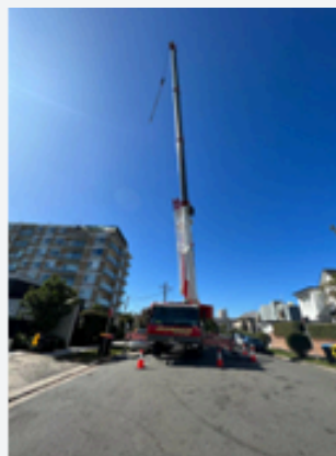
Strata re-roof, Canberra
