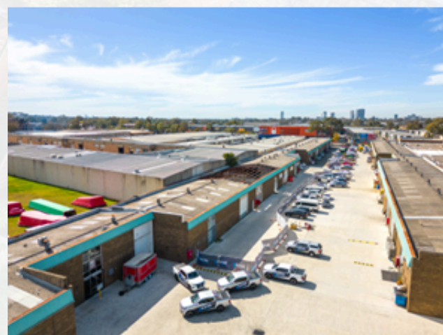
Warehouse fire rebuild, Prestons
